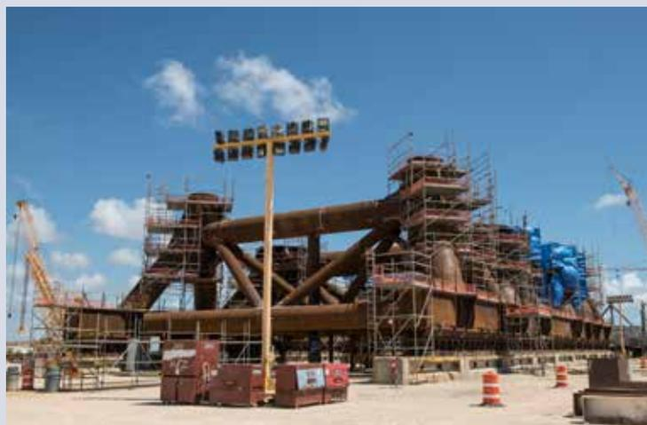
The load-out support frame is the temporary foundation for the topsides during construction in Ingleside and transport on the barge and heavy transport vessel. It is designed to fit in the 'slot' of the *Pioneering Spirit* and will be left on the barge once the topsides are picked up for final transport to field.
