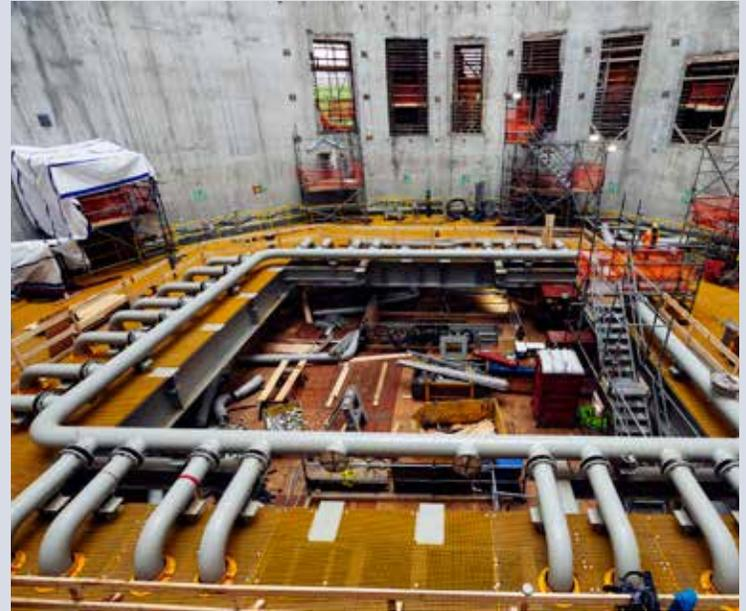
Installation of the interior decks enables more internal outfitting of the CGS. The ballast system will be used to partially flood the interior of the CGS with water, lowering it for transportation to the White Rose field, where it will be completely flooded and installed in the field.
