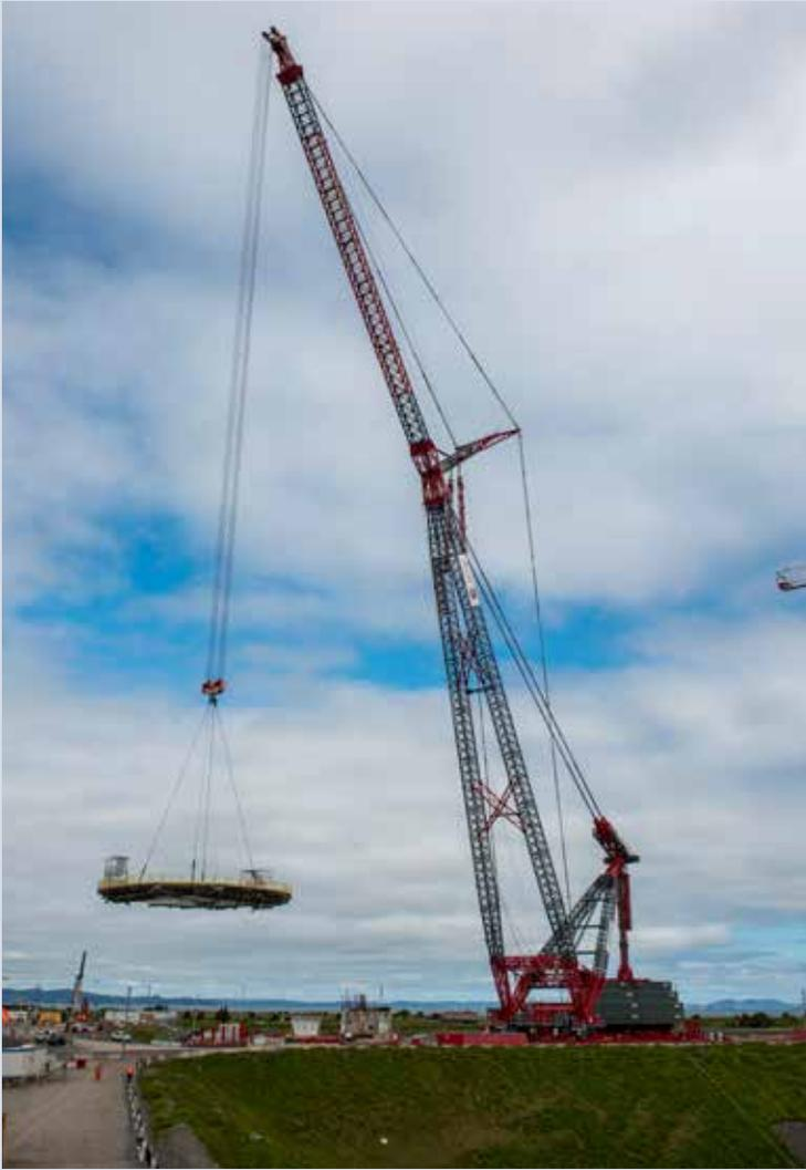
The ALE SK350 crane was officially put to work on July 12th when the first of seven interior decks was lifted into the CGS. Each deck is 174 tonnes and is carried more than 200 metres from the assembly yard on site to the interior of the CGS.
