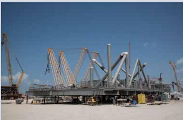
Zone 1 of the topsides cellar deck. Plate steel is transformed into I-beams and box girders on site. Each of these topsides decks is constructed in three separate pieces to ensure fit in the paint shop, then "floated" via cranes into final position within the topsides.
