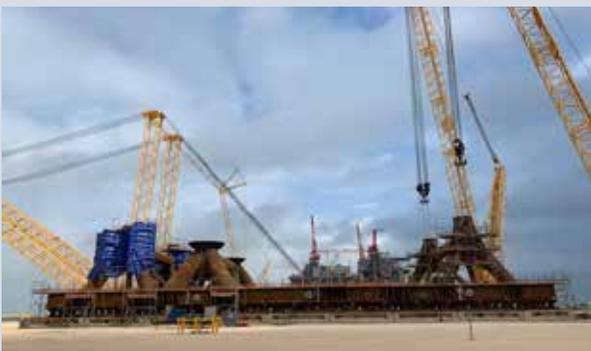
Expected to be completed construction later this year, the LSF will eventually weigh 2,263 tonnes and will carry the completed topsides. The topsides will be constructed on top, and the LSF will then be loaded on a barge for transport to NL waters.
