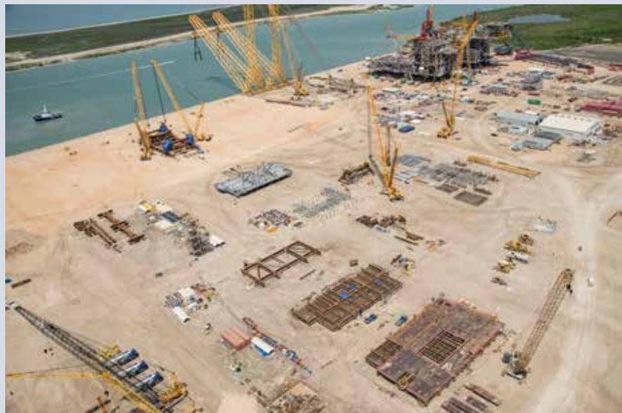
Various zones of the topsides being assembled in the Ingleside Yard. At the top of the photo, next to the water, is the load-out support frame or LSF.
