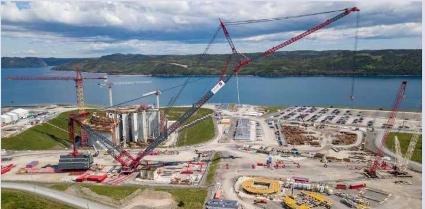
SK-350 crane, dwarfing the 46m high concrete gravity structure in the Argentia Graving Dock.
