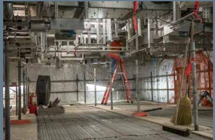
HVAC installation. A temporary floor is installed so workers can safely access the ceiling.
