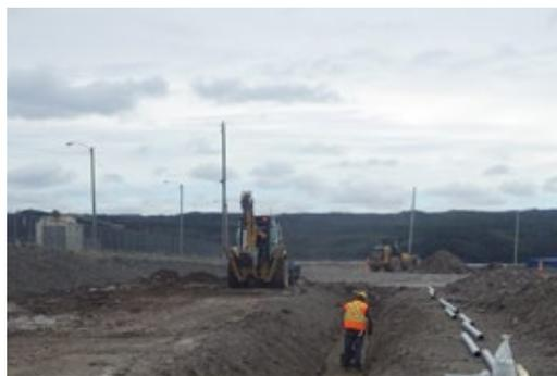
Work is picking up speed at the Argentia graving dock site. Before any concrete is poured, infrastructure has to be put in place: offices, plants, lunch rooms, and more. Above, a worker installs electrical conduits for future buildings on site.
